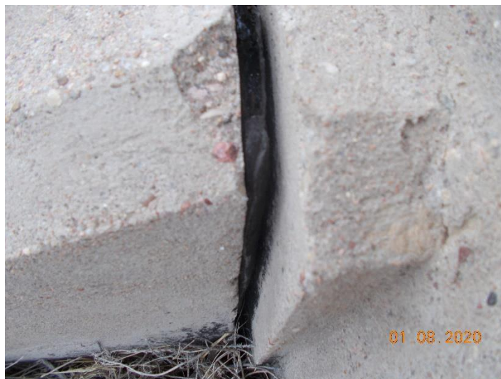
Suspect asbestos-containing material M-21-C-EJM01. The expansion joint material is non-detect for asbestos.
