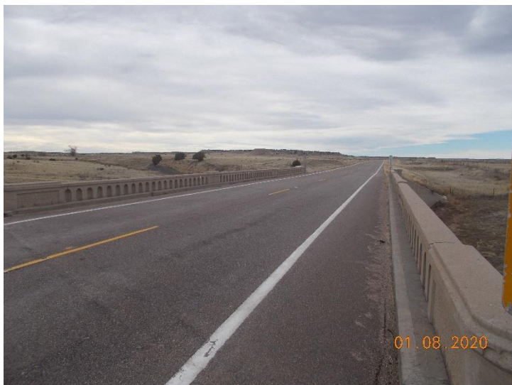
View of bridge M-21-C looking northeast.
